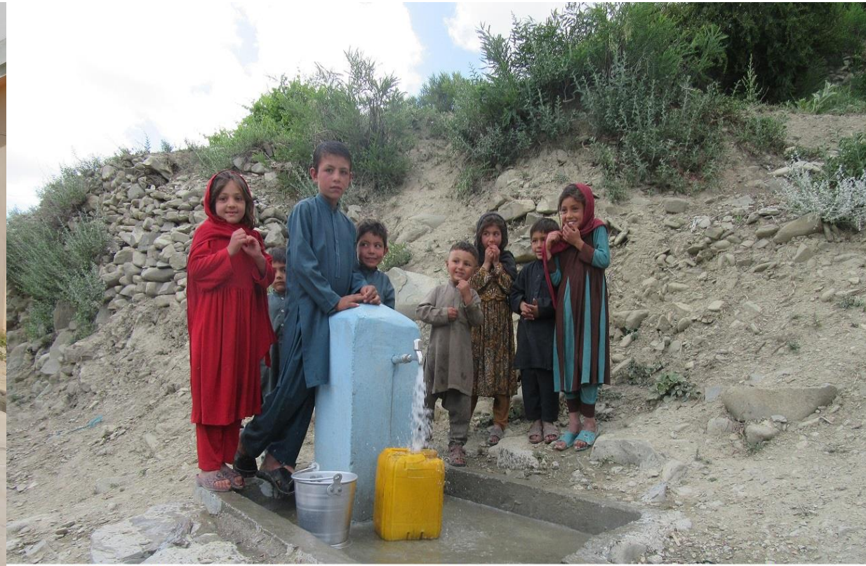
Children taking water to their homes from a newly built Water Supply Network in Ghoran village
